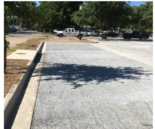
Parking lot at Alley D
